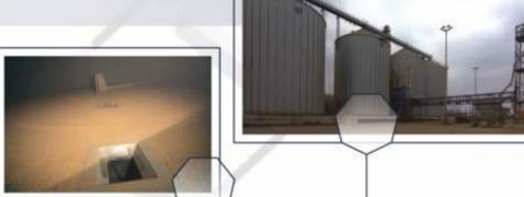
Since 2009 modern silos operate in our terminal - 4 steel tanks equipped with completely computerised system managing loading and unloading, cooperating with two electronic scales. The new system enables trans-shipment on average of 300 tonnes of commodity per hour.
